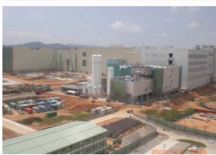
North West corner
